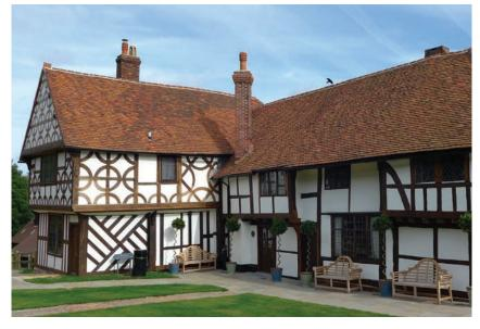
plaster infill had been replaced inappropriately in brick and concrete in the past. New panels were constructed with wood, wool and lime render to allow the building to breathe.
